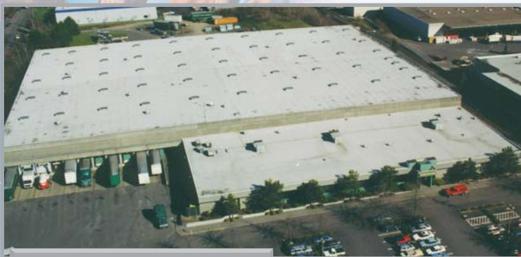
Platt Electric facility in Beaverton, Oregon.
